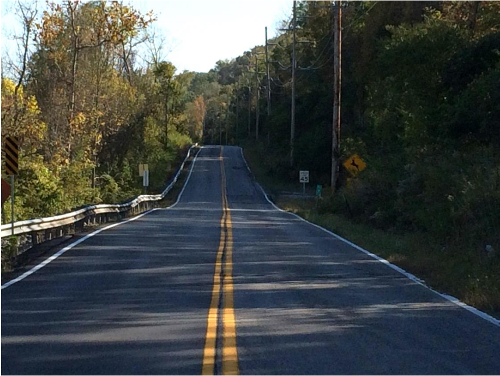
Figure 4: Southbound KY 8 near Milepost 7.0
