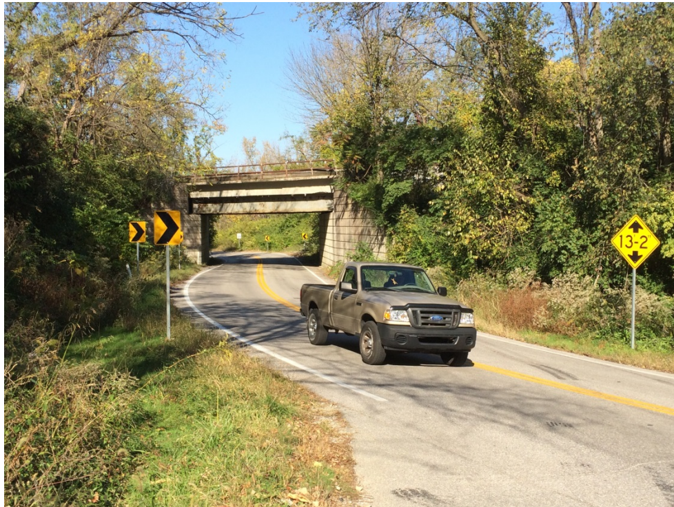
Figure 10: CSX Railroad Underpass near MP 5.0 and Tower Hill Road
