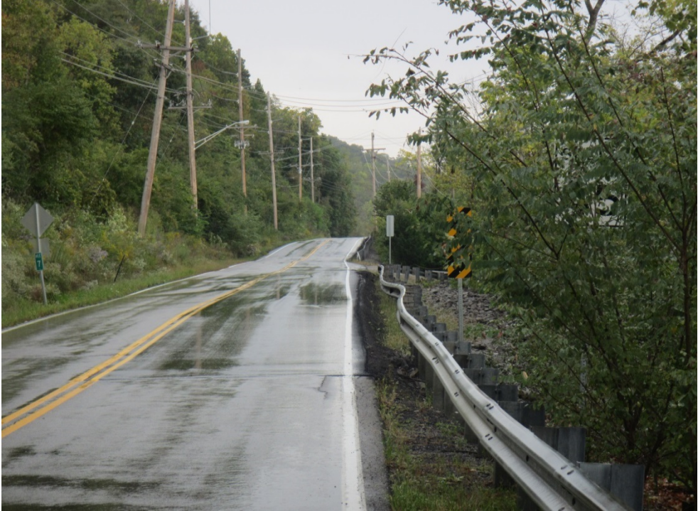
Figure 5: Northbound KY 8 near Milepost 7.0
